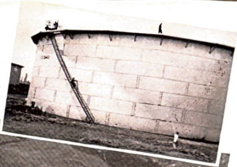
Large storage tanks are "strapped" to determine their exact capacity.
