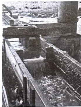
ABOVE: Taken at the Santa Fe Springs Waste Water Disposal plant, this picture shows the concrete tanks in which the oil is drained off the water. This plant handles all waste water produced by the wells in the Santa Fe and Montebello areas. LEFT: Waste water as it enters the plant.
