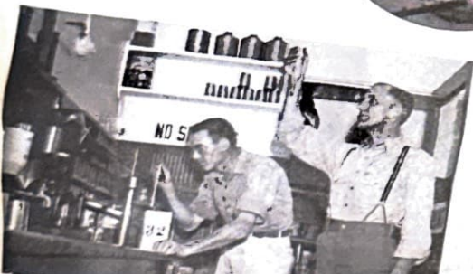
Gaugers, Clifford Perry and Hugh Jones, test crude oil samples drawn from the shipping tanks. They are provided with a field laboratory for this purpose.
