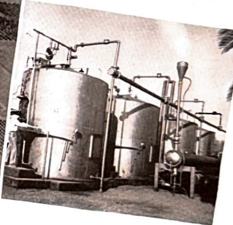
If the water content is too great, crude oil must be dried in this battery of electric dehydrators, located at the Stewart Pump Station.
