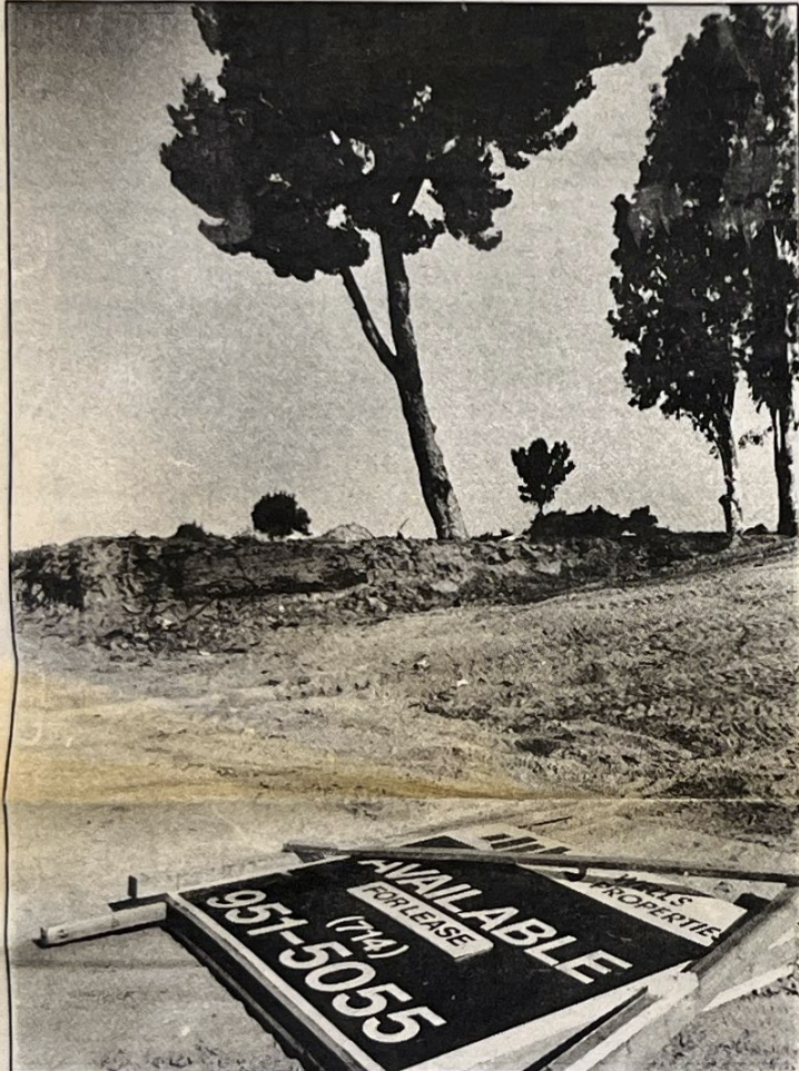
IT'S GONE — The 69-year-old Sievers-Durkee house that stood at the corner of Berry Street and Imperial Highway was leveled last week after last-ditch efforts to save the local landmark fizzled out.
