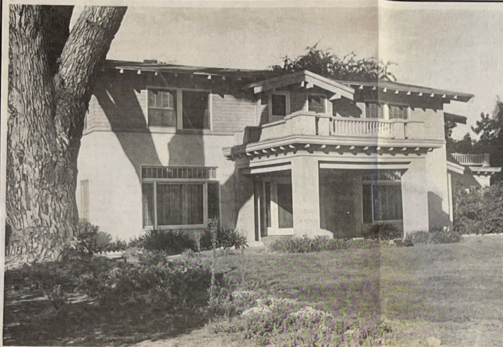
SLATED FOR DEMOLITION — The Sievers-Durkee home will be demolished Tuesday unless a solution for moving the home can be reached today. Located at Berry Street and Imperial Highway
