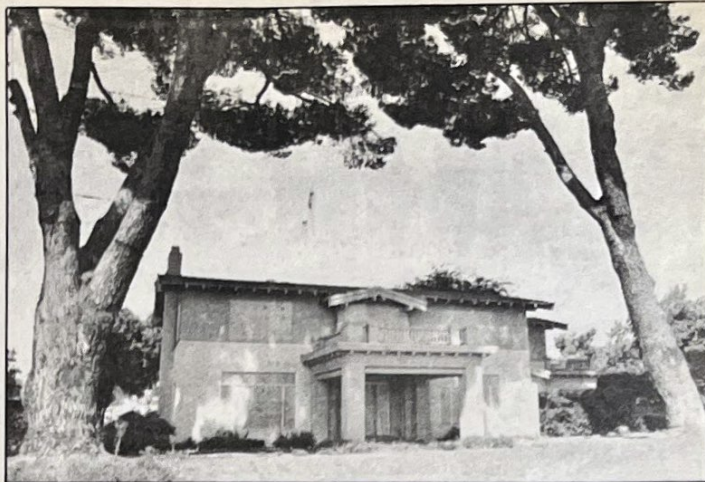
LAST LOOK? — The venerable Durkee-Bell house on the corner of Imperial Highway and Berry Street, will soon be demolished to make room for a parking lot.
