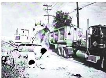
Construction activity continues.
