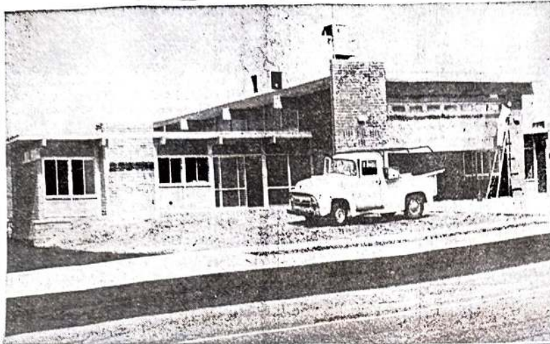
NEW BREA FIRE HEADQUARTERS ON BERRY STREET RECEIVES LAST TOUCH OF PAINT Move-in date to be set by City Council at Monday night's meeting.
