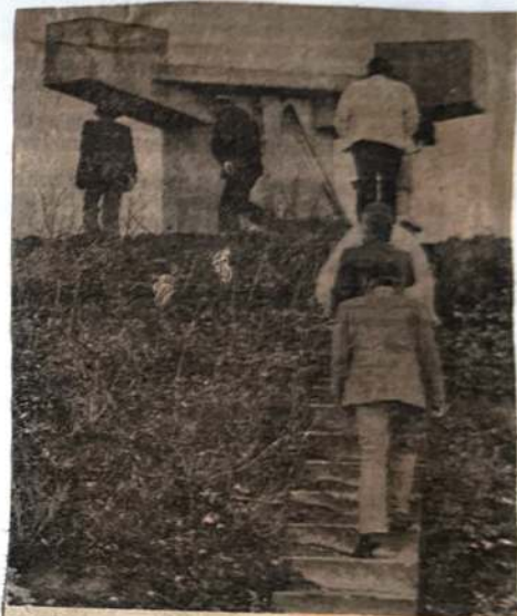
LAST TIME AROUND —Persons attending park ceremony climb steps to inspect foundation for a radar installation before structure is demolished.
