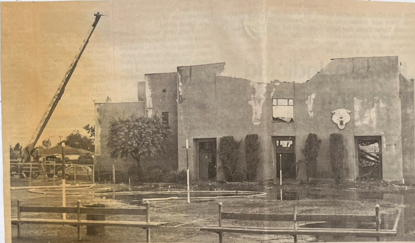
(Star-Progress photo by Stan Bird)
