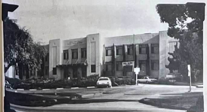
included the removal of pillars in the front of the building. At right, the school is shown as it appears now. As plans for the new facility move forward, the old structure's days are numbered.
