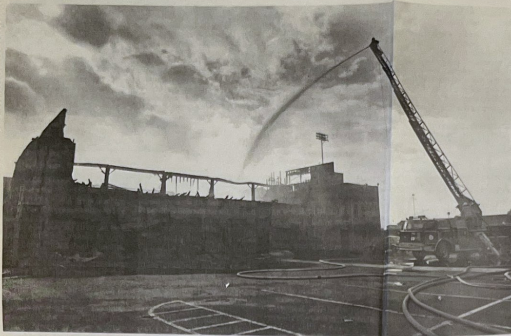
THE AFTERMATH — The remains of the Brea-Olinda High School girls' gymnasium smolders after a fire gutted the structure late
