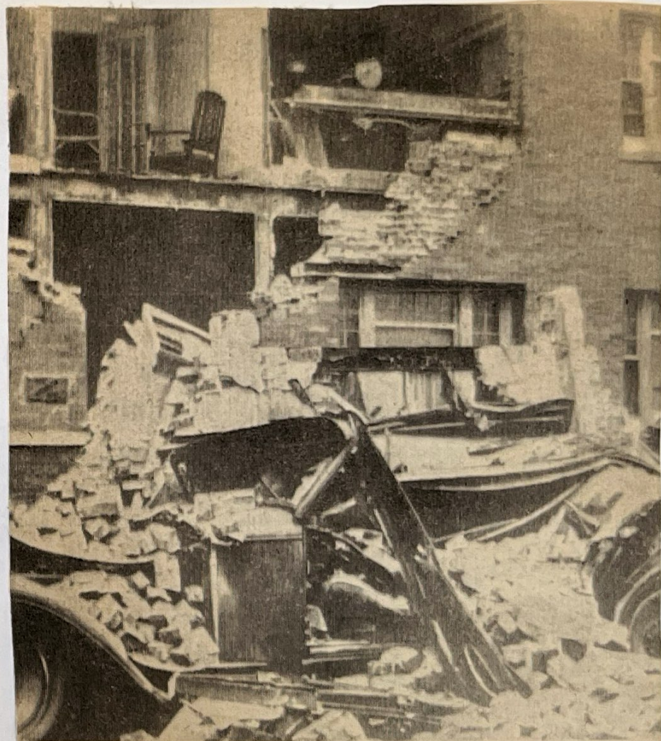
EARTHQUAKE — The March 10, 1933, earthquake, the most severe in Southland history, leveled
