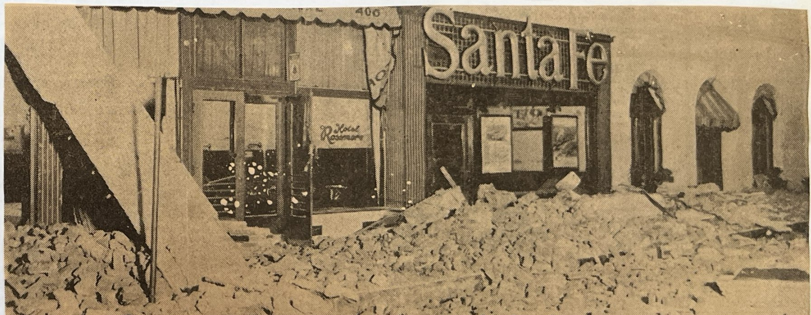
TWO DIED HERE — Mr. and Mrs. Jesse Ellison, Oakland, had checked in at the Rossmore Hotel, 403 N. Sycamore, a few hours before the quake struck. Walking out the door of the hotel cafeteria, they were crushed under tons of concrete and brick sent tumbling by the first shock that struck at 5:55 p.m. (Register photo)
