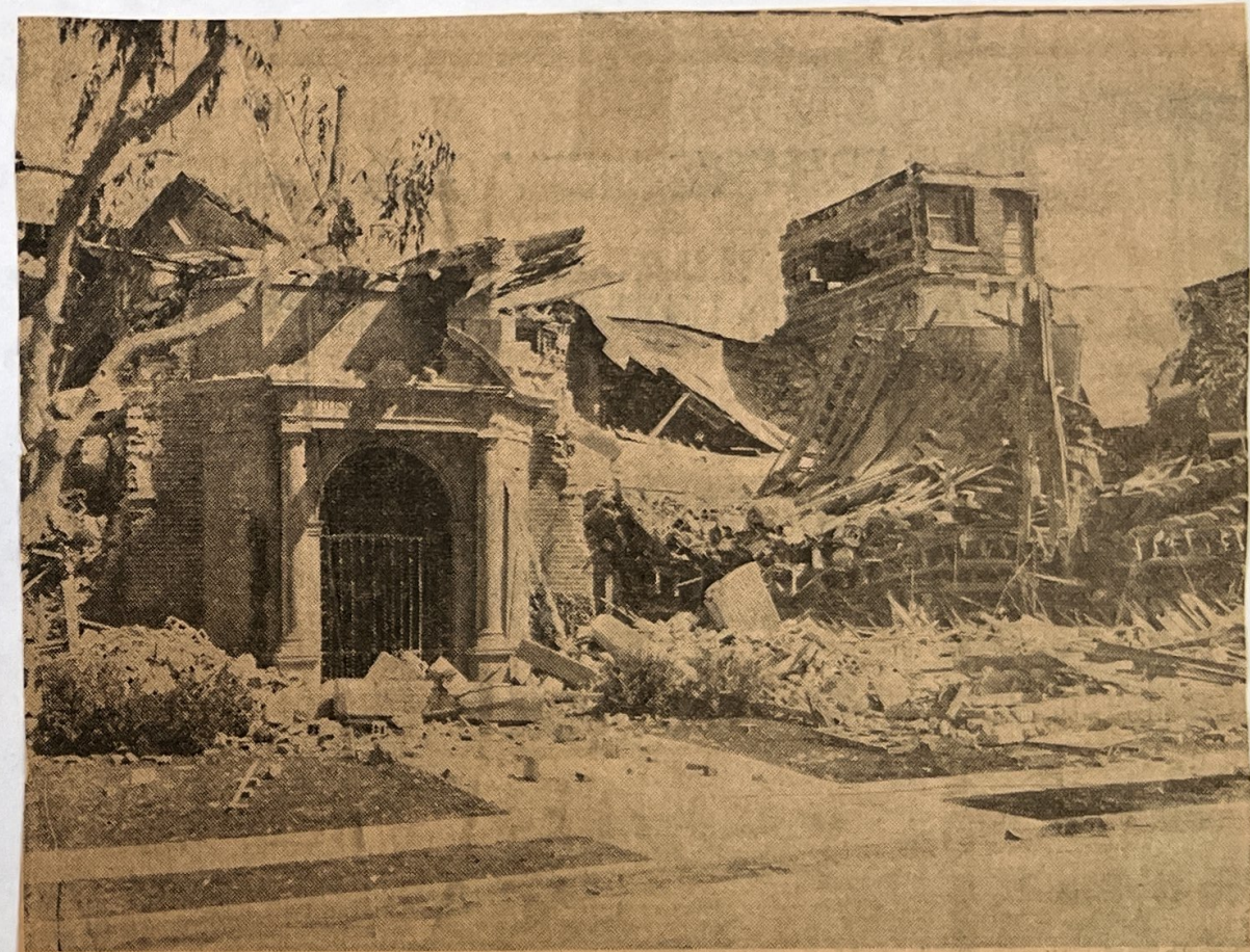
SCHOOL WAS OUT —Fortunately this school was out when Long Beach was rattled by a quake on March 10, 1933. Severe damage to schools was
