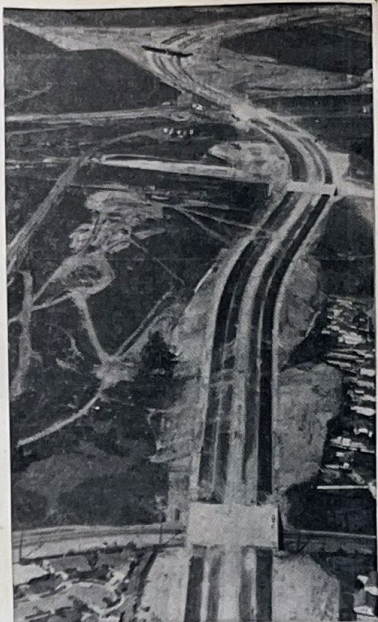
ORANGE FREEWAY — This aerial photograph gives a good look at the Orange Freeway as its heads north into the City of Brea. A new stretch of the freeway, the first in the city, is scheduled to be opened in June.
