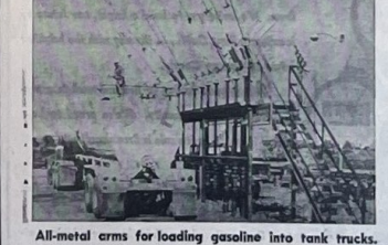
All-metal arms for loading gasoline into tank trucks.
