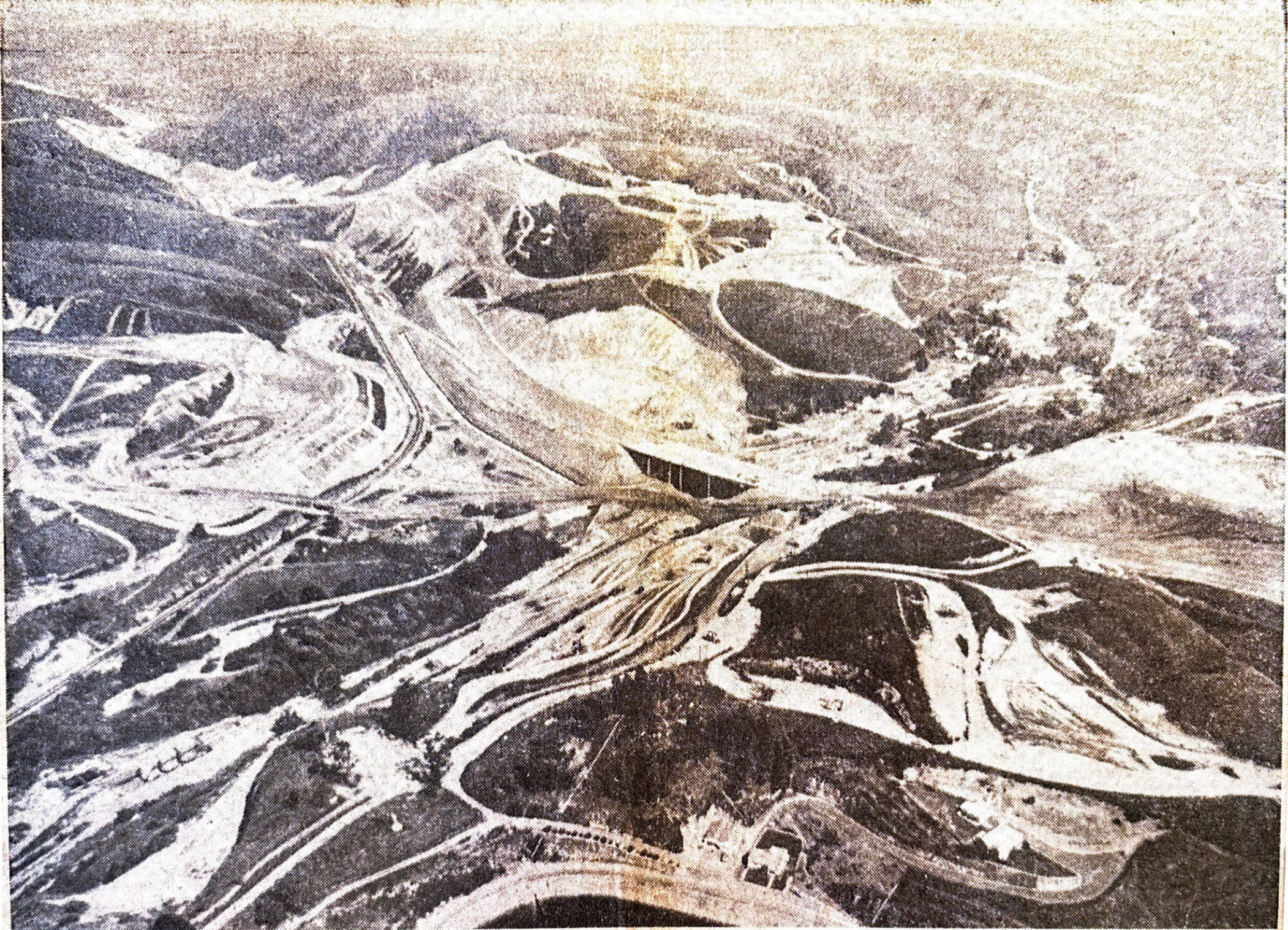
RESHAPING OF CANYON —Aerial photo shows how face of Brea Canyon is changing as segment of Orange Freeway is being constructed.
