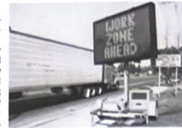
Message signs will keep Imperial Highway travelers up-to-date on construction activities.
