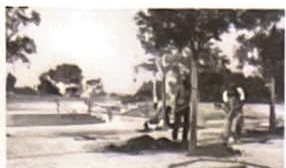
Workers apply the finishing touches on Aravista Park.
