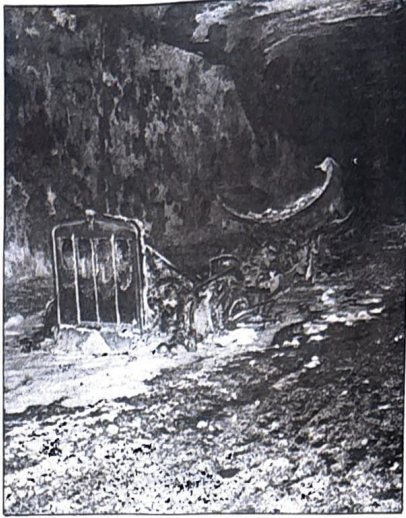
Radiator is all that's recognizable from tanker truck in tunnel.
