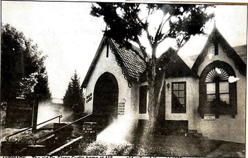
LANDMARK—The old Dr. Glenn Curtis home at 418 S. Brea Blvd. has been transformed from a crumbly
