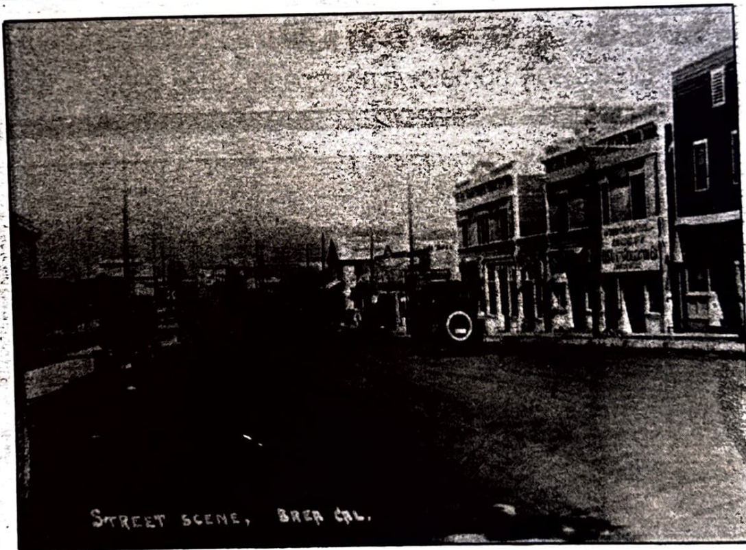
Brea reflections: Looking north from the intersection of Ash Street and Brea Boulevard, one could see this Brea street scene daily in and around 1919.
