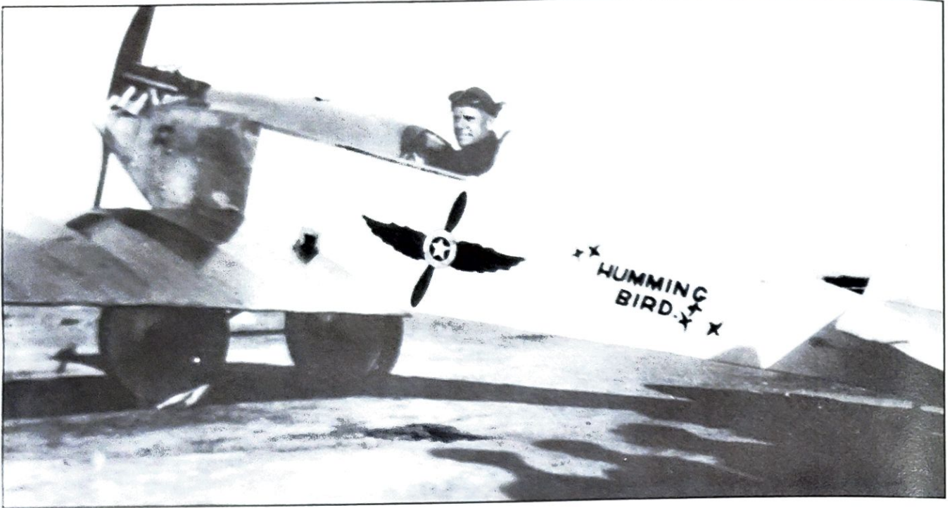
The famous Little "Hummingbird" at the Brea airport. Designed by Fred Thaheld in the Trimaine garage on Brea Blvd. In 1924 it was the first low-winged monoplane built in the U.S.A.
