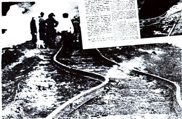
PACIFIC ELECTRIC RAILROAD tracks reduced to twisted ribbons of steel by heat from fire.
