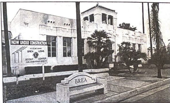
Jack E. Hancock/Brea Progress
