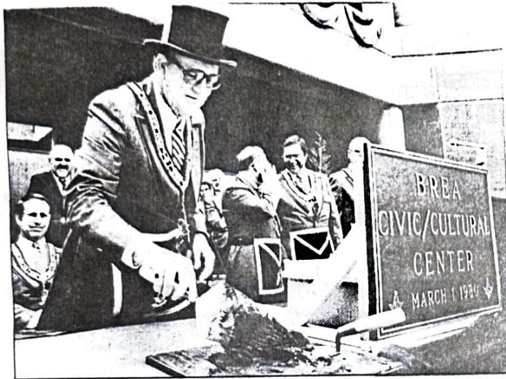
CEREMONIAL - mixing of mortar to hold the corner stone of the Brea Civic/Cultural Center is mixed by Mason Grand Master, Vernon L. Gordon. (News-Times photo by Rod Boren)
