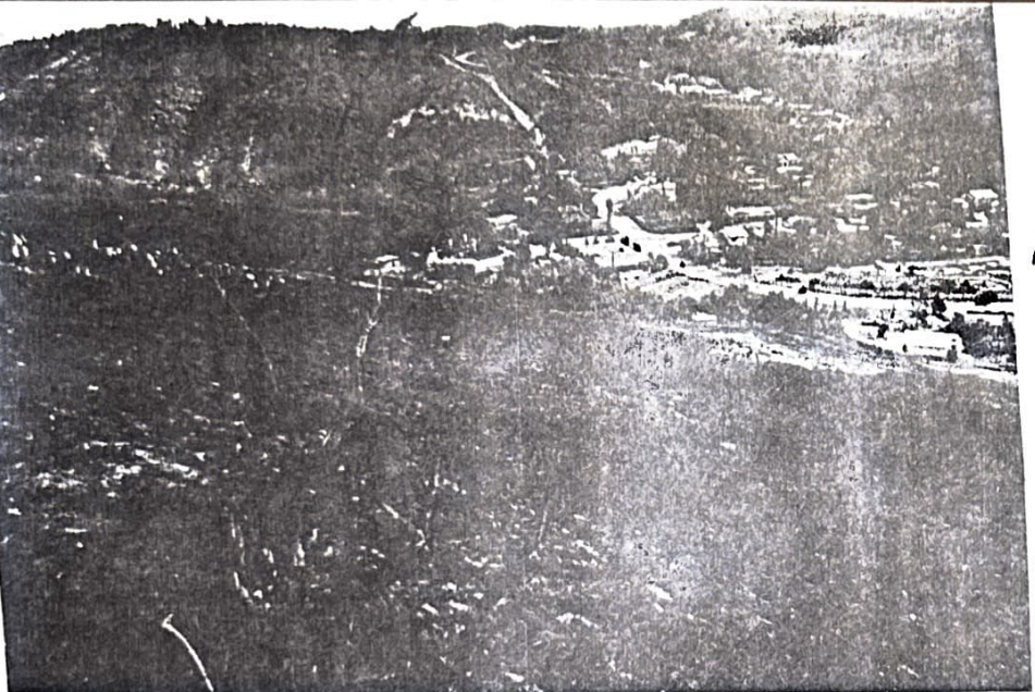
AFTERMATH OF FIRE
