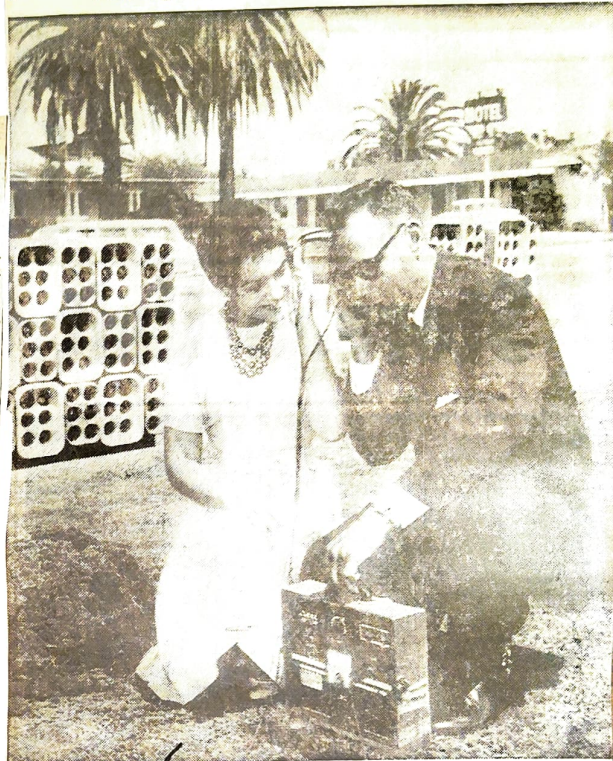
PIPE LOCATER — Pipe-locating instrument is explained to Pacific Telephone's Louise Rickner by engineer Al Kellam. With the mecha-
