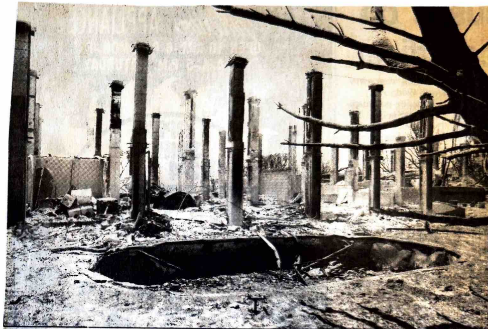
IN THE WAKE OF DISASTER — Charred columns stand amid the rubble of an 8,000-square-foot mansion ravaged by Wednesday's Carbon Canyon fire that claimed many homes in Sleepy Hollow.
