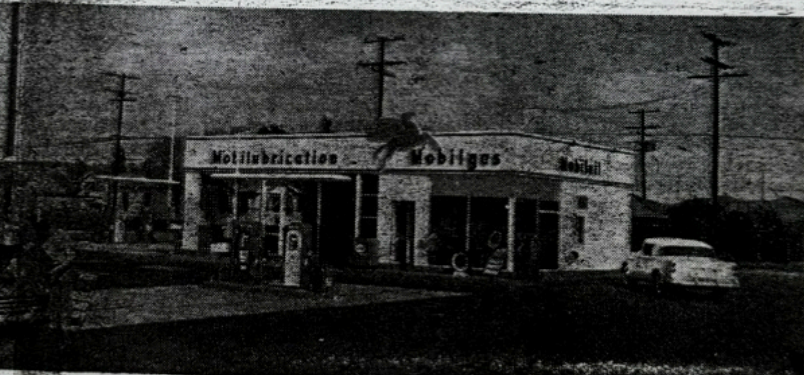
Grand opening of the modern, six-pump Mobilgas Station shown above is being staged this Friday, Saturday and Sunday at the corner of Pomona Avenue and Elm Street. The station is being operated by a native of Brea, Dale Varnar. There will be free gifts for adults and kids during the opening celebration.
