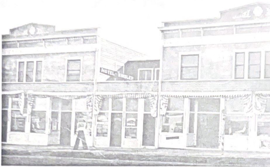
Hotel Kinsler between the movie theater and pool hall. ca. 1922
