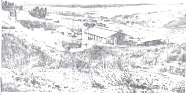
• This is the original refinery and water cooling tower used by the Brea and Birch oil companies
